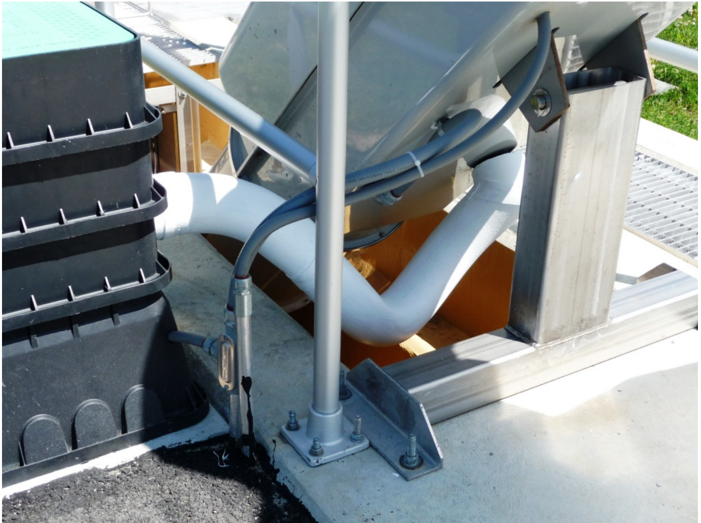
(Insulated Water Supply Line)
