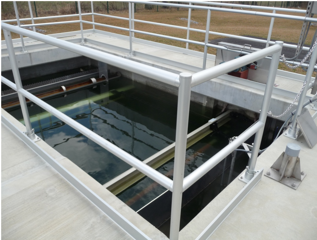
Bethel WWTP (above)
