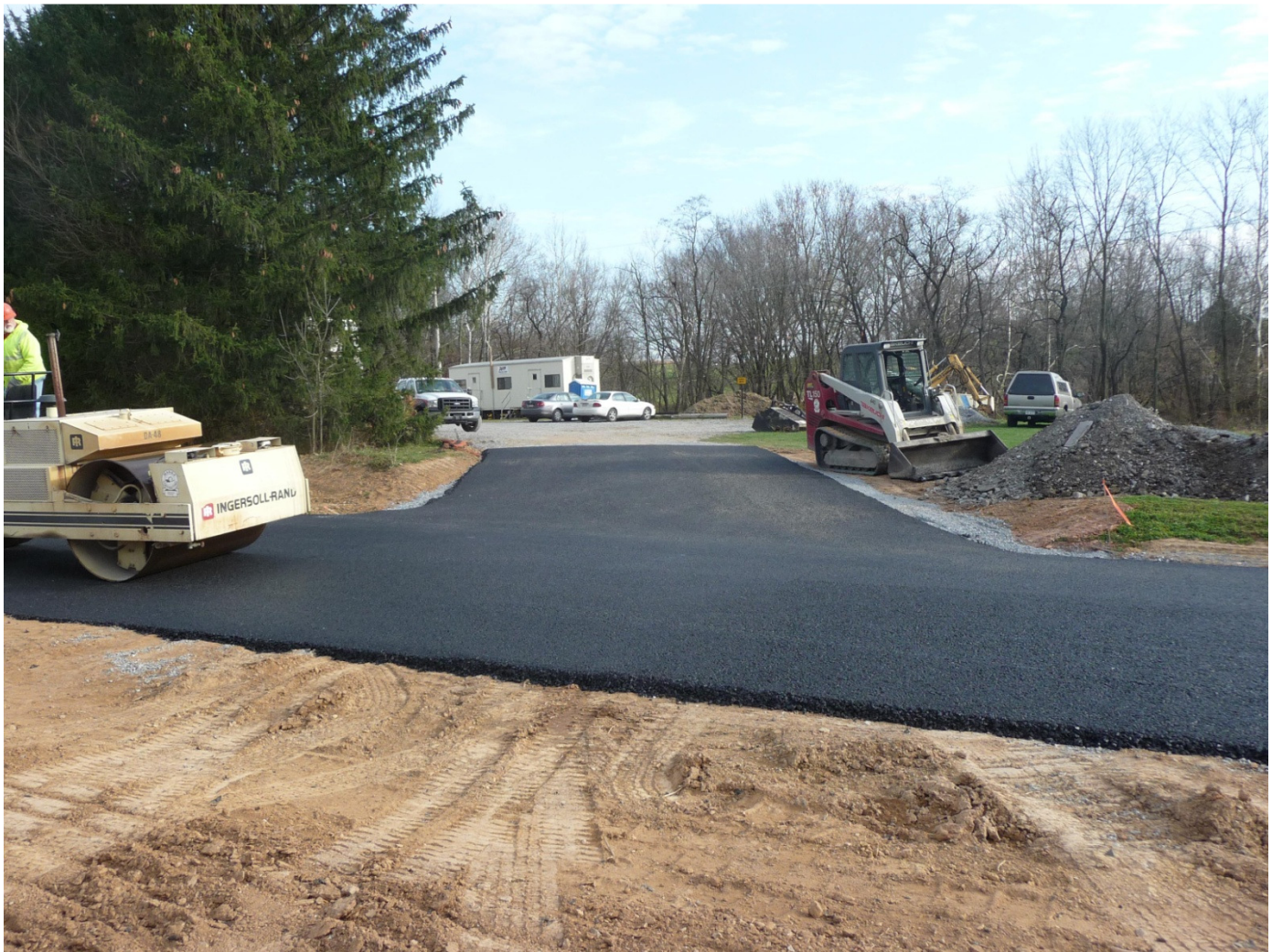
Bituminous Binder Course Placement at Driveway to Fzystown WWTP
