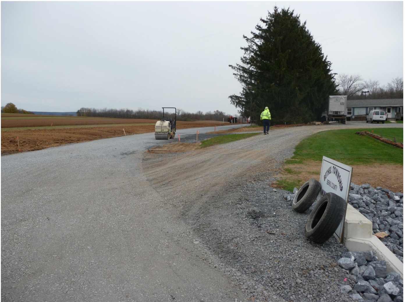
Frystown Waste Water Treatment Plant Driveway Entrance
