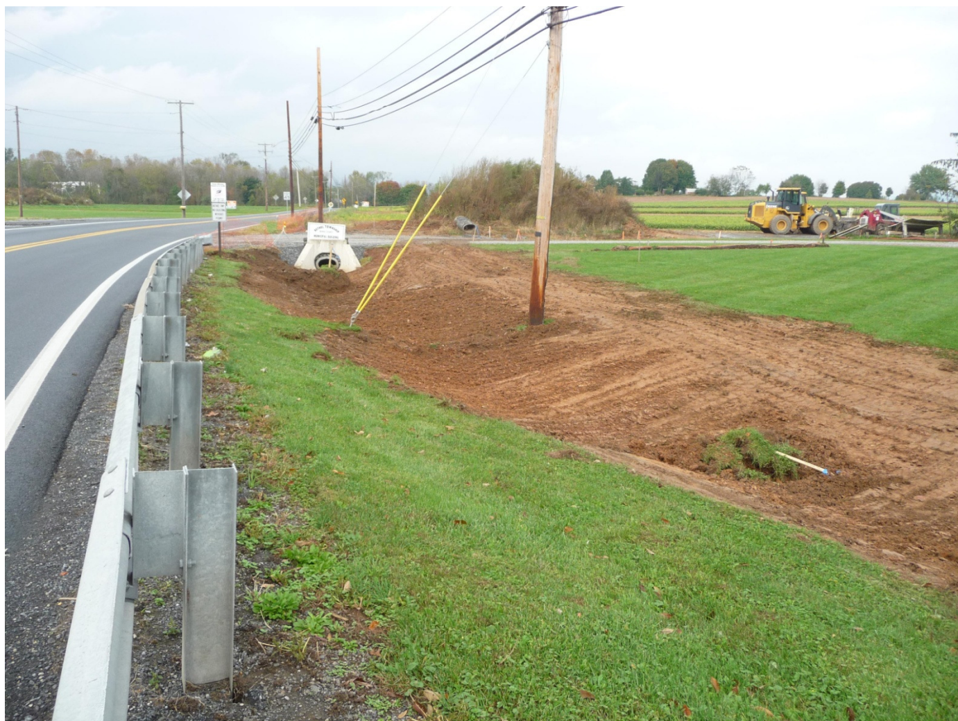
Swale Construction along Camp Swatara Road near the Driveway to Frystown WWTP
