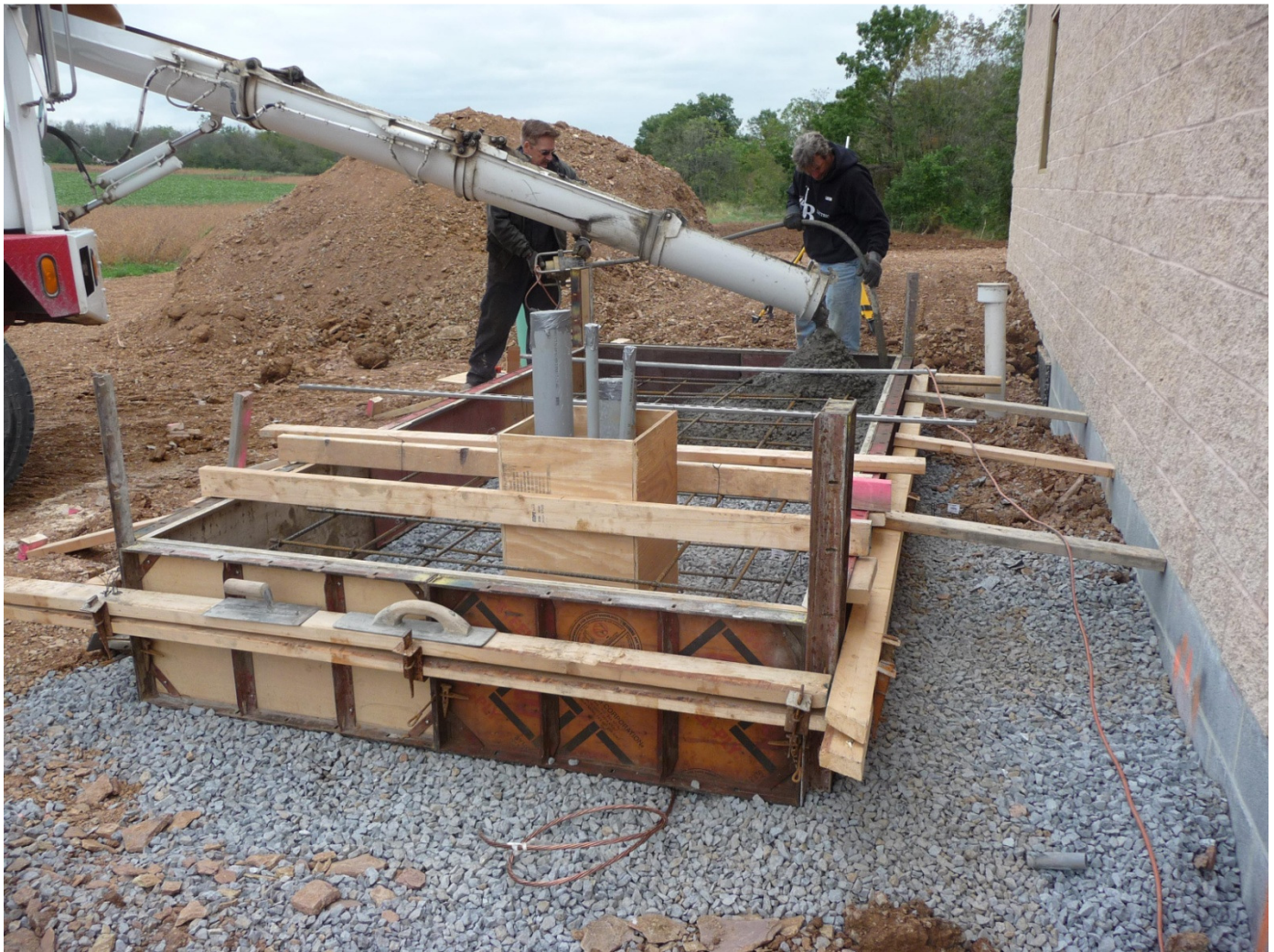
Concrete Placement for Generator Pad Outside of Frystown WWTP Control Building
